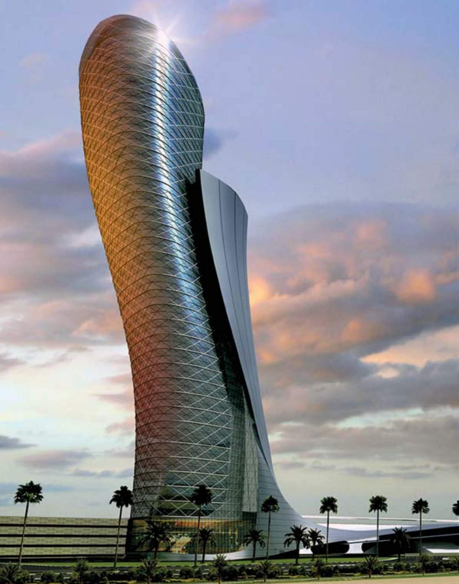
Capital Gate - Abu Dhabi (United Arab Emirates)
