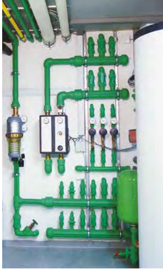
Distribution network for domestic water and heating in residential buildings
