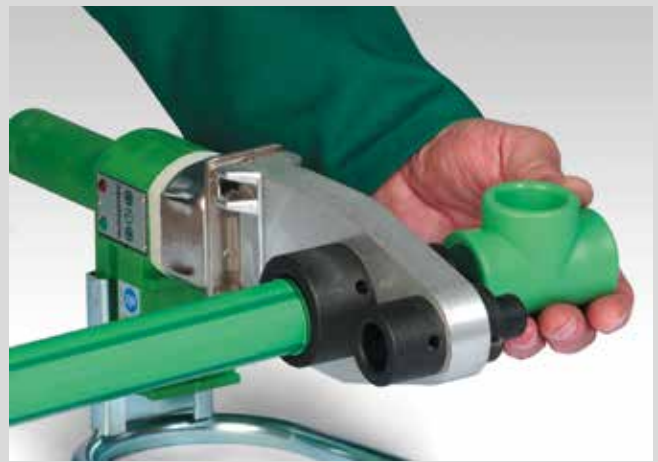
Heating-up of pipe and fitting
