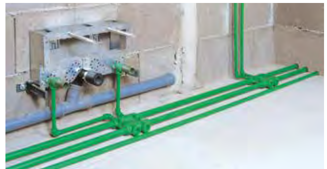
Floor distribution with distribution blocks
