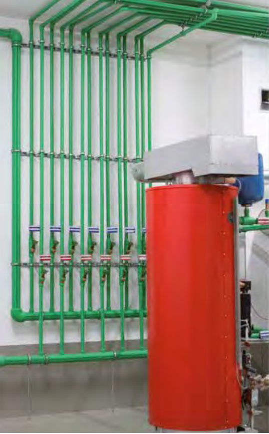
Distribution network for domestic water and heating in residential buildings
