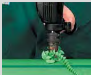
Drilling through the pipe wall
