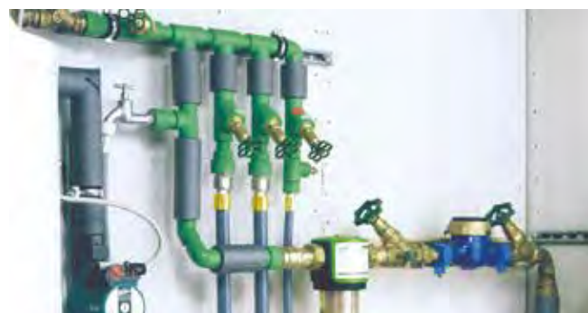
House connection station
